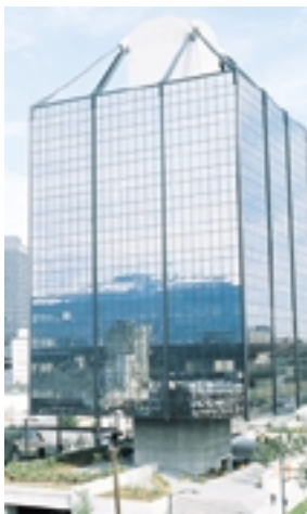
Figure 5.55 This office building in Vancouver is specially built so that it will not collapse in an earthquake. The floors are suspended from the central core of the building by huge cables that are visible at the top. What do you think will happen to this building when the ground moves in an earthquake?
