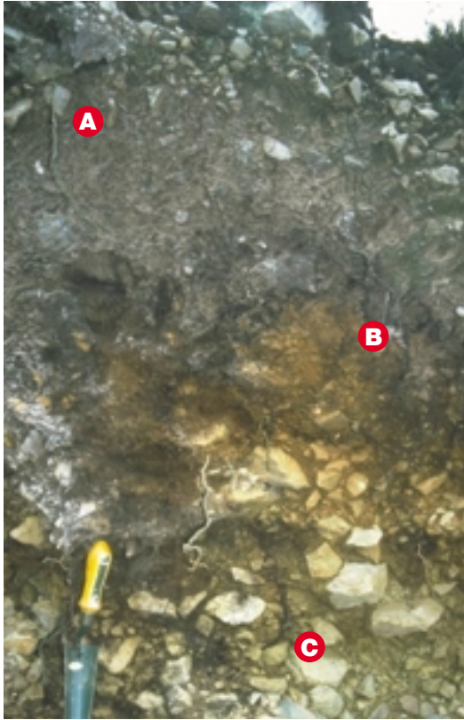
Figure 5.22 Exposed soil profile of an eroded hillside
