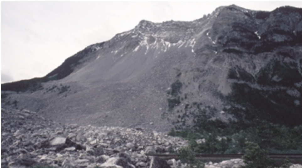
Figure 5.31 The most disastrous rock slide in Canadian history was the Frank Slide in 1903 in Alberta’s Crowsnest Pass. Over 80 million tonnes of rock crashed down the side of Turtle Mountain, burying part of the town of Frank. More than 70 people died in the disaster. The slide lasted less than 100 s. Scientists are studying the Frank Slide using new technology and sound waves.
