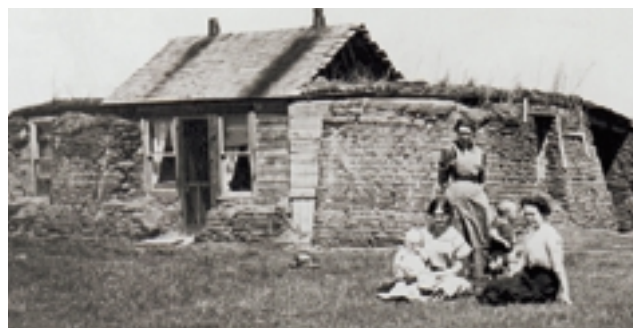
Figure 3.1F Sod houses provided protection from the weather, and the soil helped to prevent heat from escaping.
