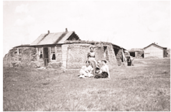
Figure 11.8 A sod house in the Camrose area of Alberta, likely about 1900. It had a dirt floor. What would be the benefits or drawbacks of raising young children in this house?
