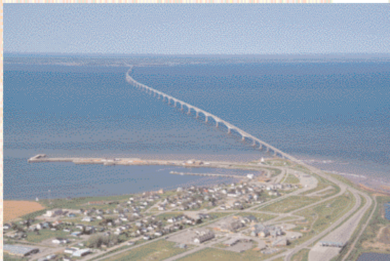
Figure 10.14 The Confederation Bridge, looking south toward New Brunswick. The promise of a link to the mainland was important to the people of PEI when they decided to join Confederation. What benefits do you think the bridge provides for PEI?
